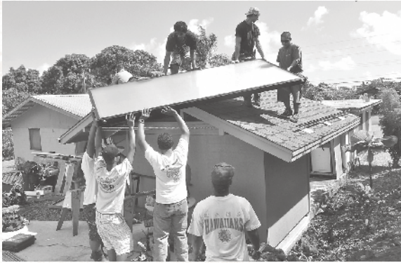
Students installing solar hot water system
